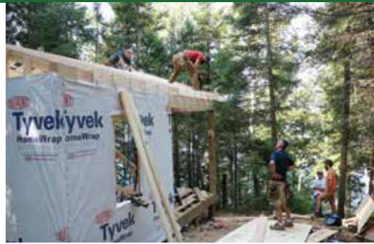
Construction continues on the Island sauna.
